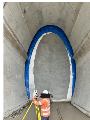
Figure 2.16: SOP Site – tunnel portal
