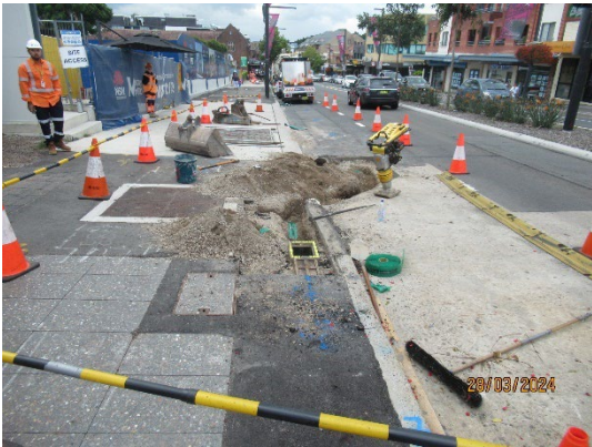
Figure 1 3 Truck turntable installed in the south entry of the Western Shaft (Five Dock).
