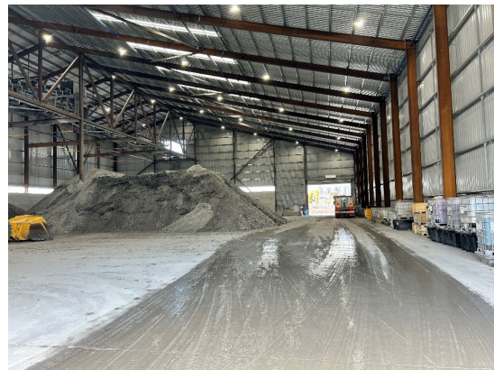
Figure 2.10: Rosehill Site – TBM Spoil shed
