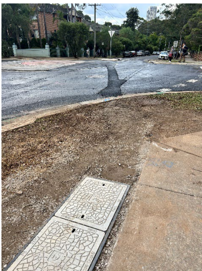
Figure 4.1: Westmead Utility Works – Cnr Hassell and Bailey Streets
