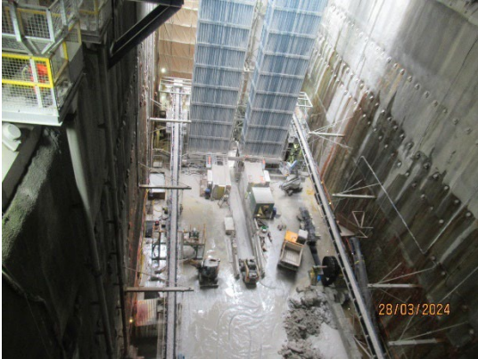
Figure 1 1 Works in the station box (The Bays).
