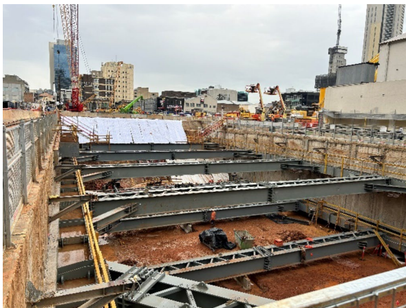
Figure 2.3: Parramatta Site – Station Box excavation
