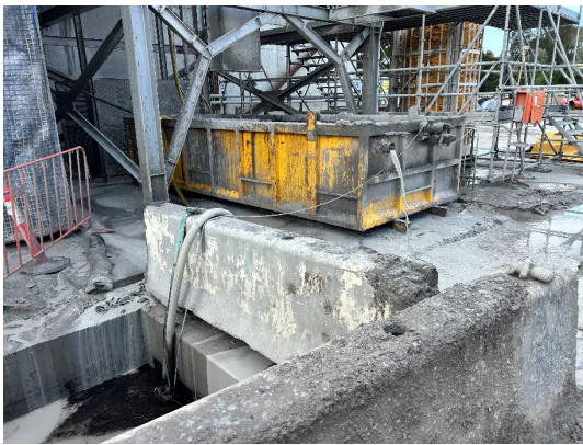
Figure 2.7: Rosehill Site – Slurry coming off TBM Spoil conveyor
