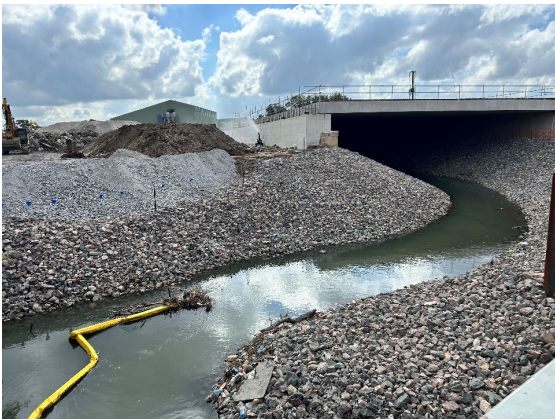
Figure 2.11: Clyde MSF Site – Parramatta Station box spoil storage at Clyde MSF
