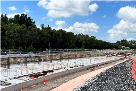
Figure 2.13: Clyde MSF Site – Utilities retaining wall construction
