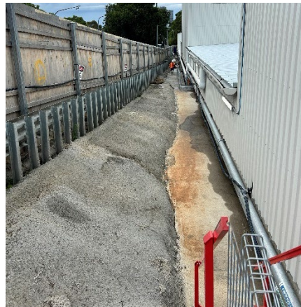
Figure 2.2: Westmead site – Clean stormwater drainage path
