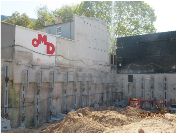
Figure 3.3 Pyrmont West: Movement of spoil to form piling pad.
