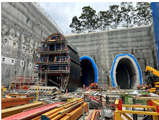
Figure 2.15: SOP Site – tunnel portal formwork construction
