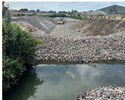
Figure 2.12 – Clyde MSF Site – A'Becketts Creek low flow construction
