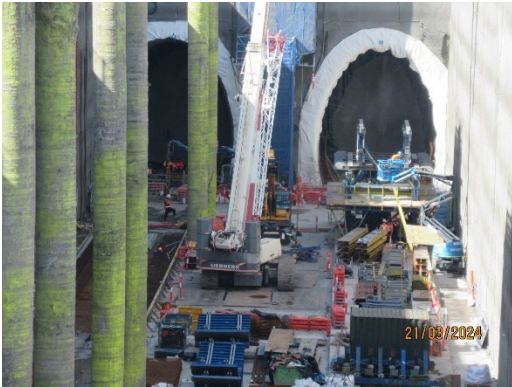
Figure 1.7 Works in the Nozzles (North Strathfield)
