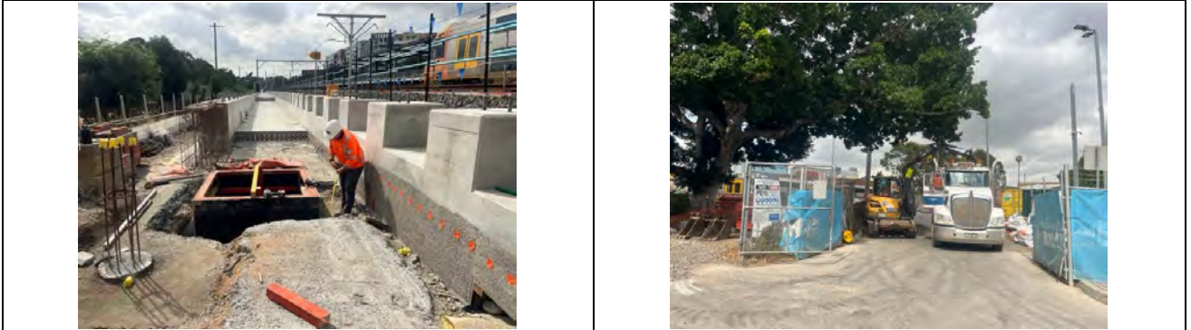
Construction of the new platform at Bankstown Station ongoing.
