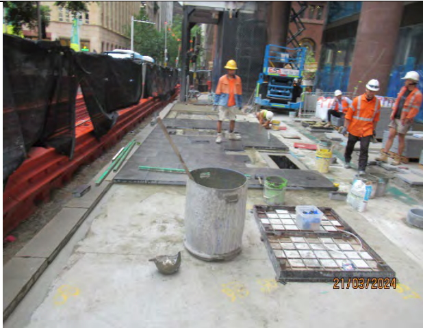
Martin Place South: Footpath tiling works.
