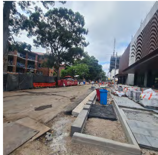
WL ISD Cope St Site Compound: Paving, kerbing, construction of rain gardens and stormwater works ongoing.
