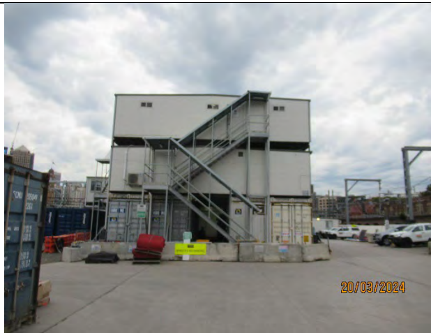
Sydney Yard: Remaining site sheds in use by Sydney Metro and LOR.
