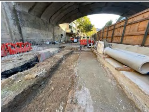
Road and pavement works ongoing in Zone 6.
