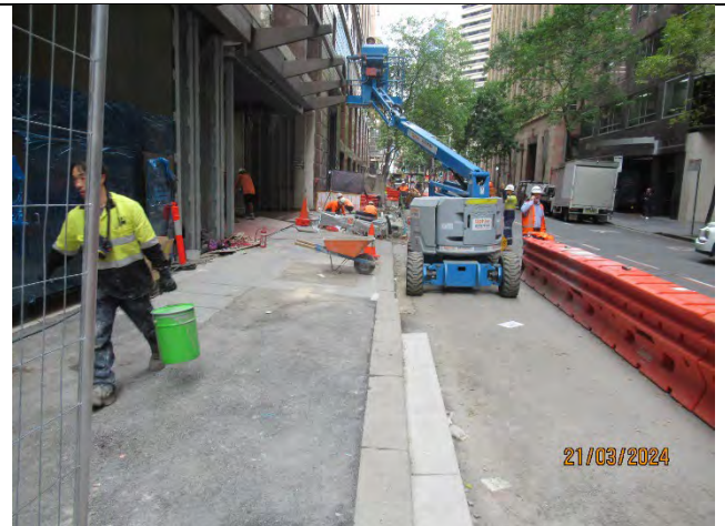
Martin Place North: Works on footpath on Castlereagh Street.
