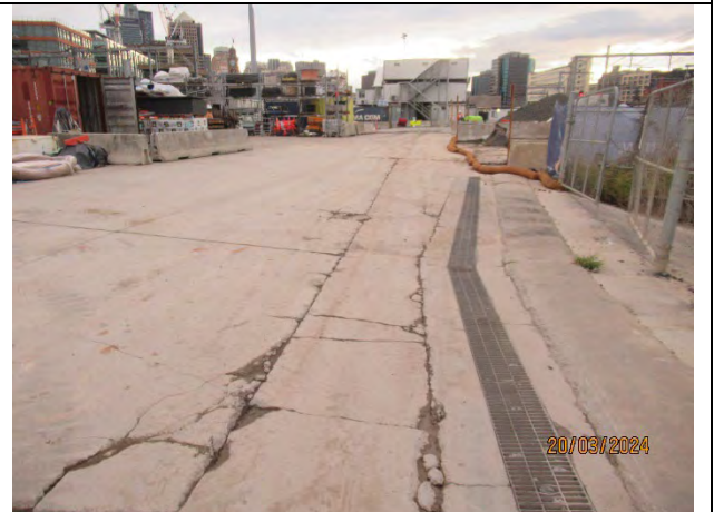
Sydney Yard North: Ongoing use of the Sydney Yard by other Sydney Train Contractors.
