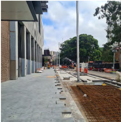
WL ISD Cope St Site Compound: Paving, kerbing, construction of rain gardens and stormwater works ongoing.
