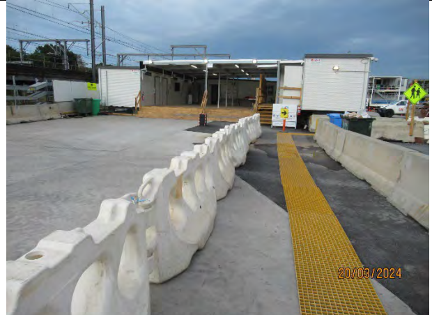
Sydney Yard: New site sheds in use by other Sydney Train contractors.
