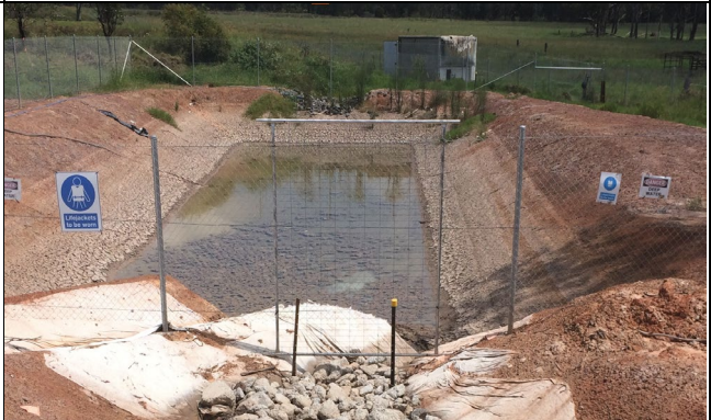
Bringelly facility – Sediment basin empty and well managed.
