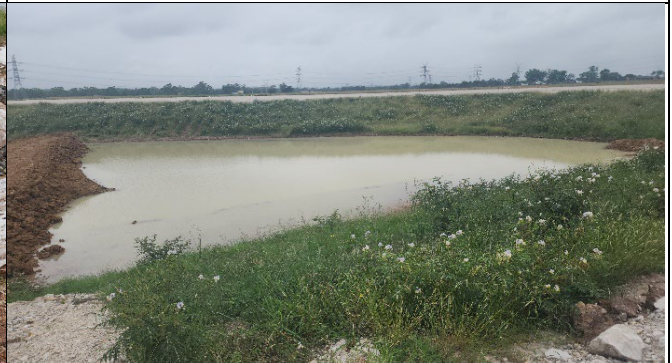
SMF – water retention basin had been constructed. It is noted that weeds required maintenance.
