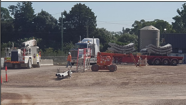
Claremont Meadows shaft view north – Tunnel segment delivery from Orchard Hills.
