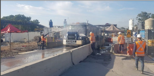
Orchard Hills – Manual truck wash following automated wheel wash.
