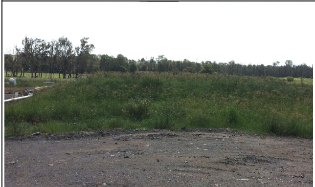
Bringelly Facility west – Weeding campaign required.
