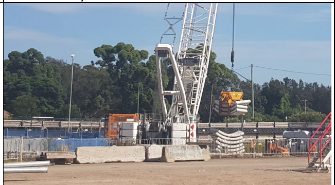
Claremont Meadows north west – Tunnel segment storage and crane to shaft.
