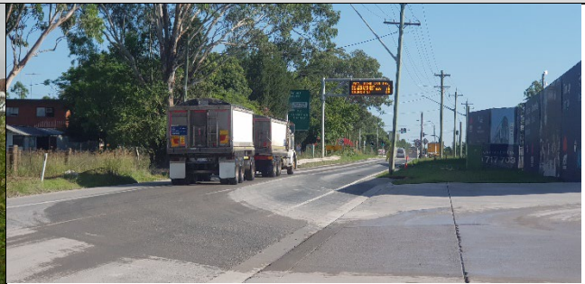
Kent road view north at site access – Suggest increasing frequency of use of water cart on the exit apron and street sweeper on internal roads.
