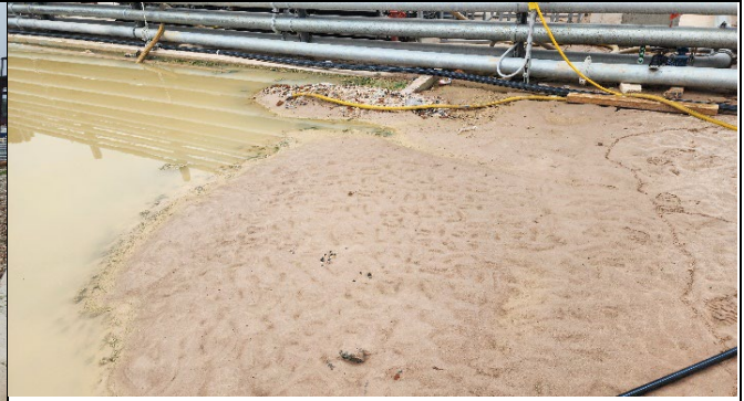
ORH – Sediment accumulation at the sump
