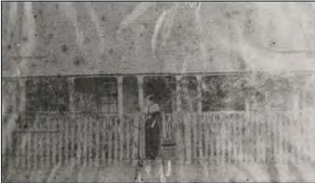
Figure 2.4 'Belrose' cottage, home of the Bryson family, ca. 1870s (Source: Picture Willoughby, File No: 003/003989).
