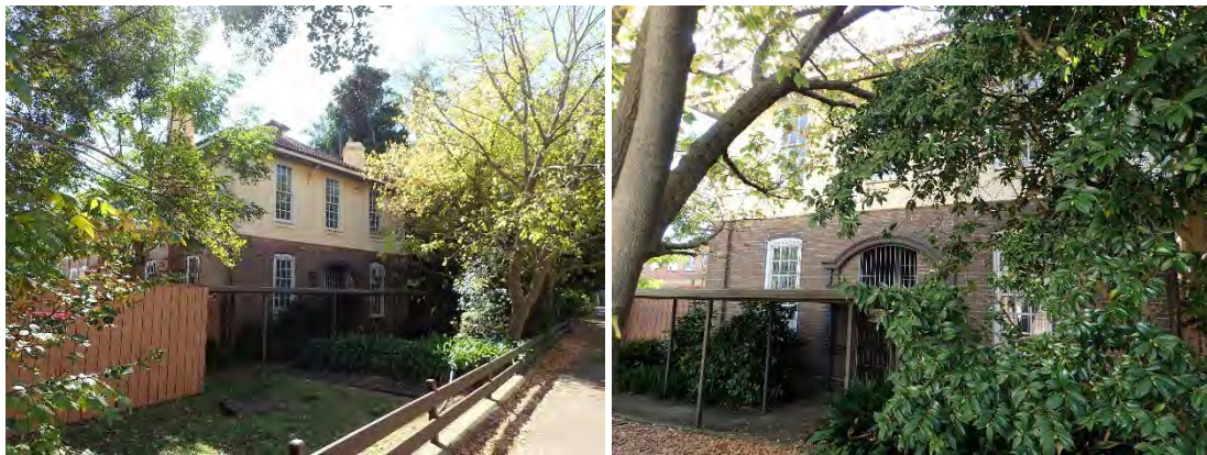
Figure 11 Two views of the southern elevation of Mowbray House in 2017. Note the intrusive porte cochère.
