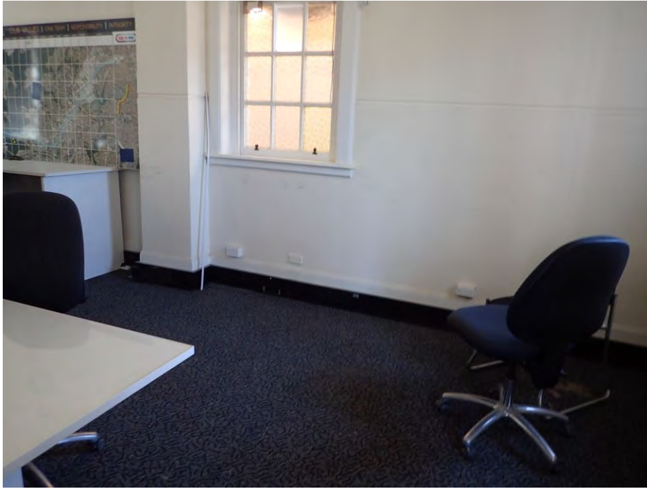
Figure 4 Existing conduit, power cable trays and sockets have been retained and painted. The windows and doors have been retained in good order and some have been re-painted.
