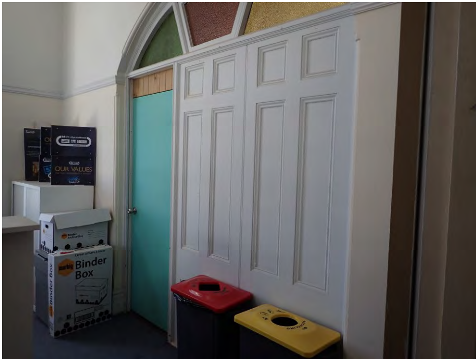
Figure 6 The missing leaf (door) from the folding door between Reception and the Mail Room has been replaced by a secure (lockable) door, which will be replaced by the original door.
