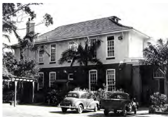
Figure 2.18 1950s view of Mowbray House School after purchase by Sydney County Council (Source: Picture Willoughby, File No: 003/003321).
