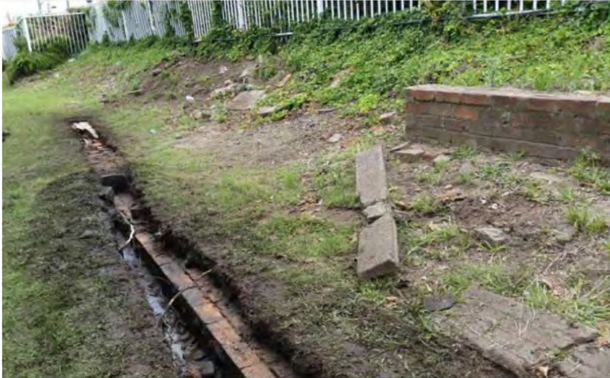
Figure 6: Platform at Hamilton Station classified as a 'work' by the project archaeologist, Wickham Transport Interchange project, 2015
