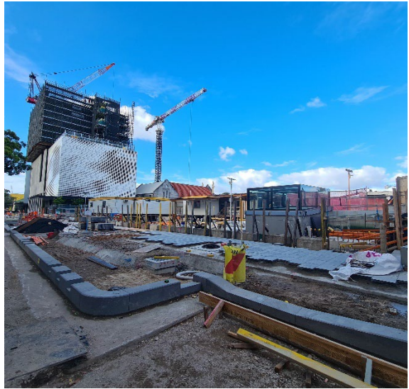
WL ISD Northern Building and Cope St Site Compound: Paving, kerbing and construction of rain gardens underway.
