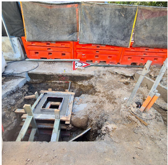
Cope St Site Compound: Stormwater pit FRP works underway.
