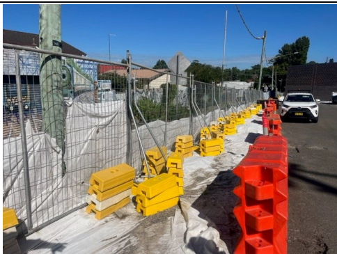
ERSED controls had been established at the Dulwich Hill MSB to reduce risk of sediment runoff. Noise mats were in place around the generator.
