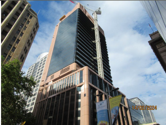
Martin Place South: View from Martin Place. Tower crane now removed.
