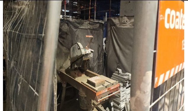
Clark Street public domain works – Pavers were cut within a noise enclosure within Site C (good practice).
