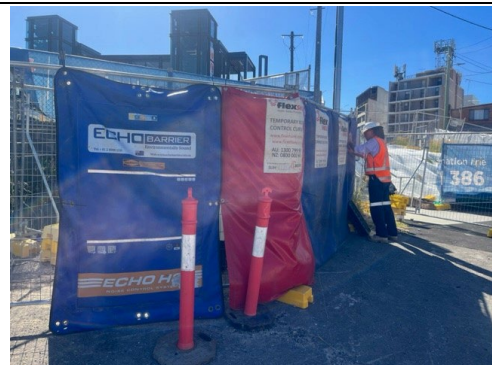
ERSED controls had been established at the Dulwich Hill MSB to reduce risk of sediment runoff. Noise mats were in place around the generator.
