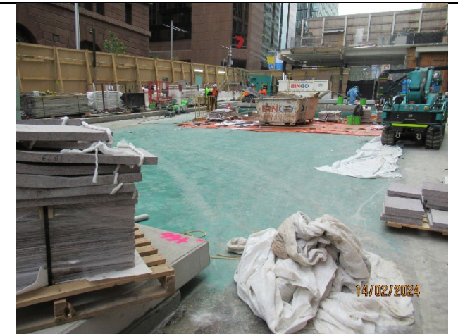
Martin Place: Works in the public area such as waterproofing.
