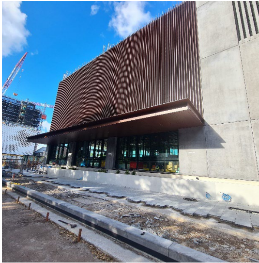
WL ISD Northern Building and Cope St Site Compound: Paving, kerbing and construction of rain gardens underway.
