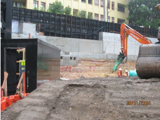
Figure 3.1 Pyrmont East: Profiling of sandstone wall beneath retaining wall.
