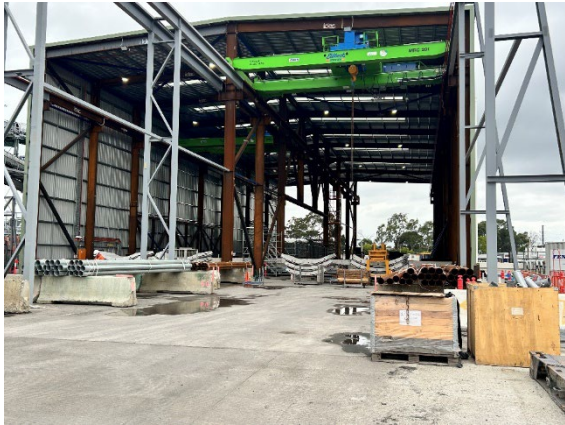
Figure 2.7: Rosehill Site – Segment Shed
