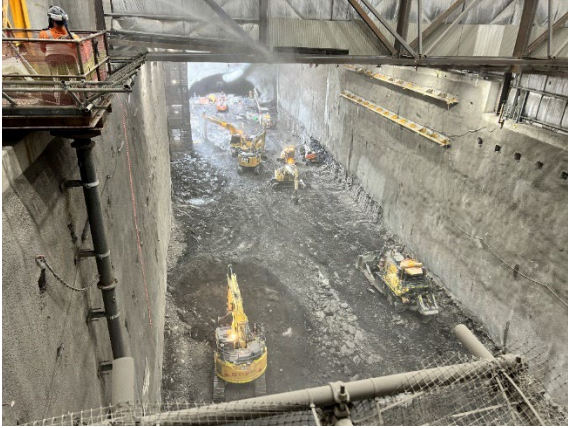
Figure 2.1: Westmead Site –Station Box excavation
