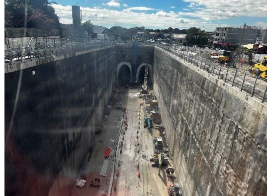
Figure 1 4 Blinding completed. Construction of TBM traverse plinths (Burwood North).
