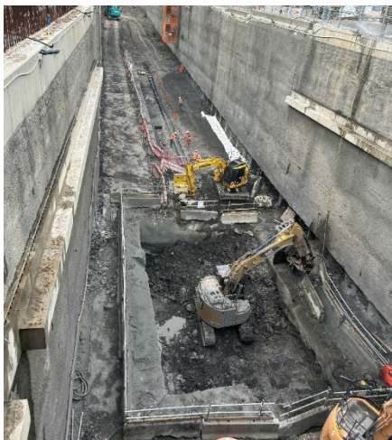
Figure 2.5: Clyde Dive site – Clyde Dive excavation continuing with rock hammer
