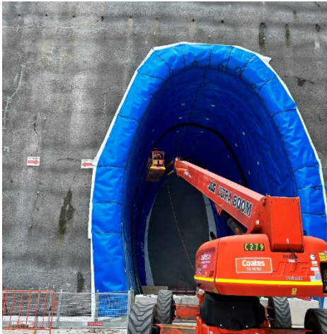
Figure 2.15: SOP Site – Caverns waterproof membrane installation
