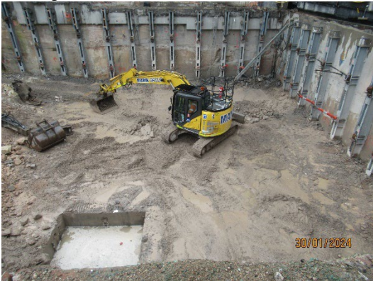
Figure 3.3 Pyrmont West: Carpark basement columns, slabs and beams removed.
