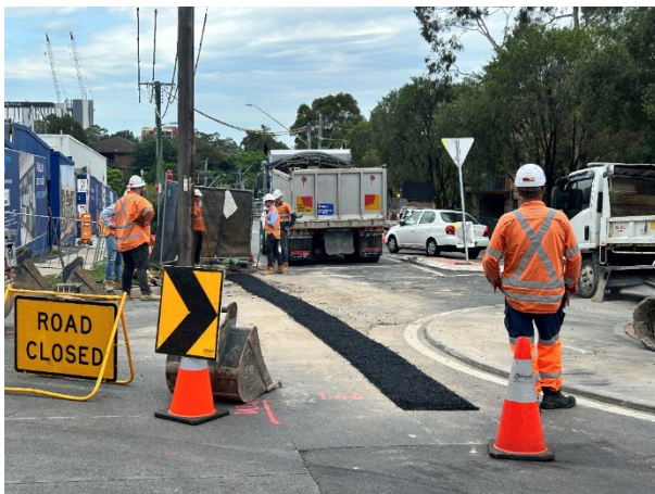
Figure 4.1: Westmead Utility Works - Bailey Street following conduit installation
