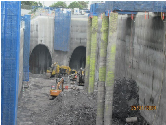
Figure 1.7 Removal of remaining spoil. Works on the Nozzles. (North Strathfield)
