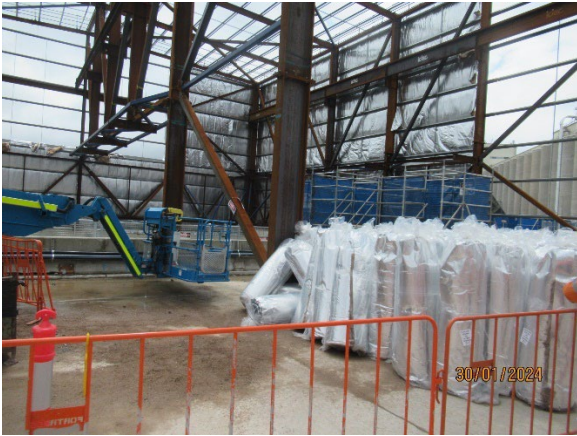
Figure 3.7 The Bays: Cladding being placed on the frame of the Segment Shed
