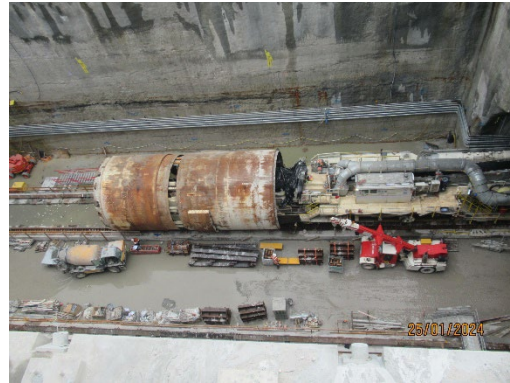
Figure 1 2 TBM in the Western Shaft (Five Dock).
