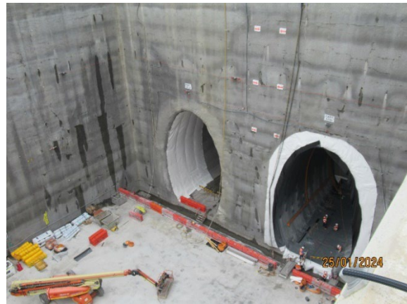
Figure 1.8 Waterproof membrane being installed in the nozzles (SOP).
