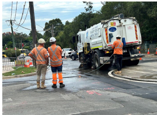
Figure 4.2 Westmead Utility Works: Noise blanket gaps during day works.
