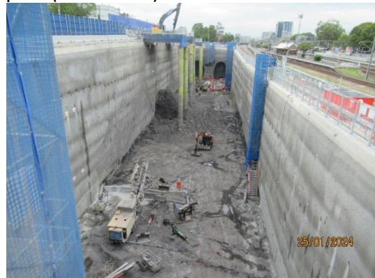
Figure 1 6 Ongoing excavation of station box and nozzles; wall support (North Strathfield).
