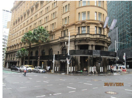
Figure 3.6 Radisson Hotel: Construction of hoarding as a safety precaution.
