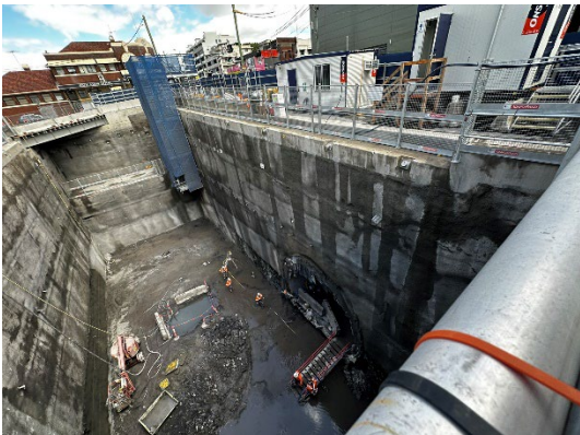
Figure 1 5 Ongoing excavation and wall support South Shaft (Burwood North).
