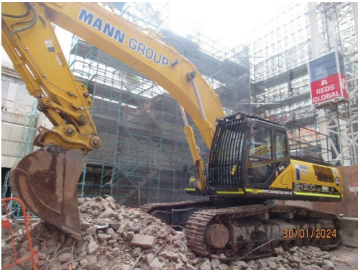
Figure 3.5 Hunter St West: Ongoing demolition on George Street
