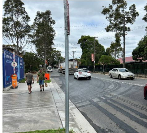
Figure 2.2: Westmead site – Hawkesbury Road Repairs completed
