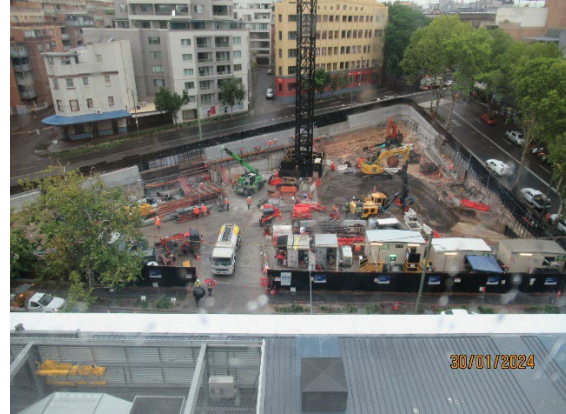
Figure 3.2 Pyrmont East: Ongoing retaining works around the boundary of the site
