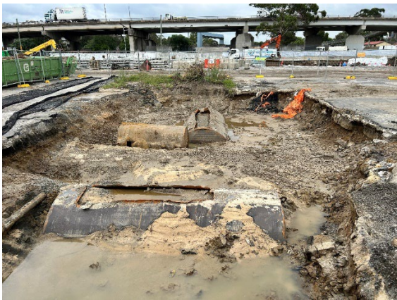
Figure 2.11: Clyde MSF Site – UST removal and remediation
