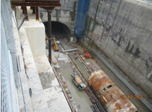
Figure 1 3 TBM Traverse through the Western Shaft (Five Dock).
