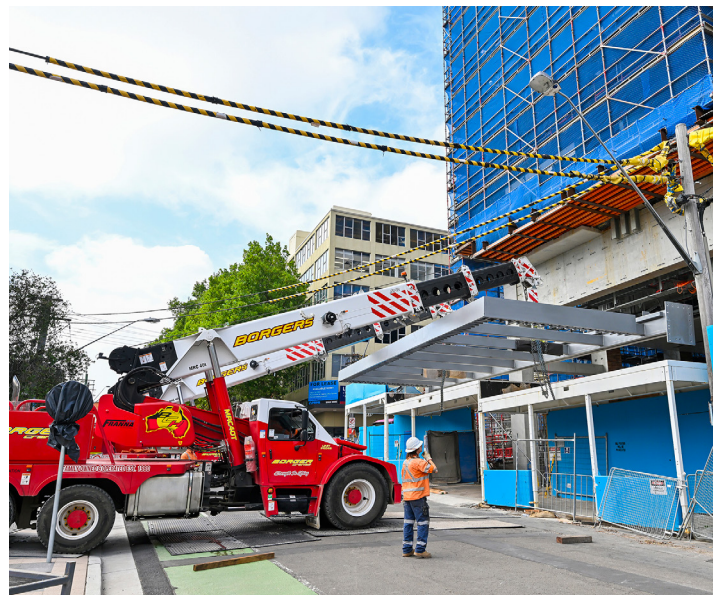
Installation of entrance awning at Clarke Street
