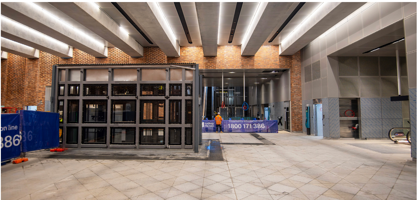
Concourse level nearing completion
