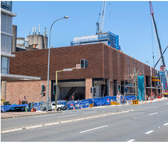
Completed brick façade work at Oxley Street and Pacific Highway
