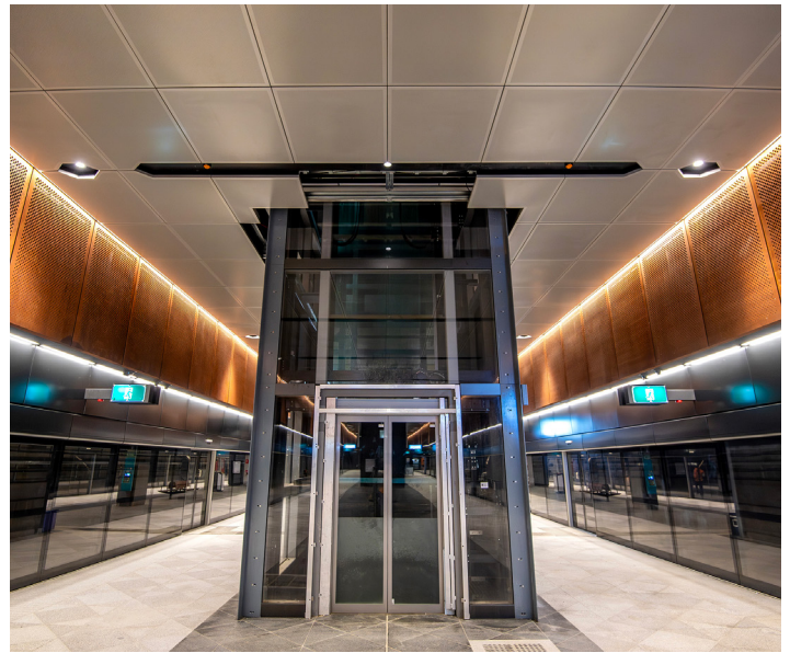
Platform lifts installed and commissioned
