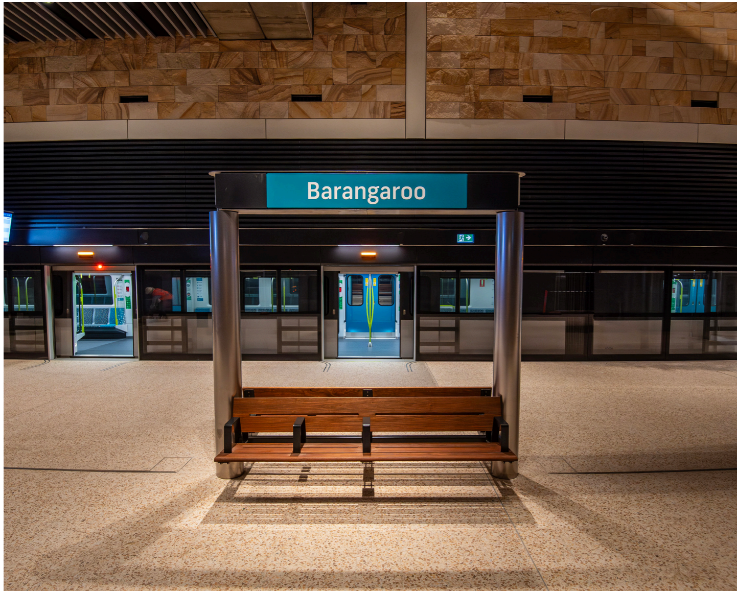
Train pulled into the platform at Barangaroo station behind platform screen doors
