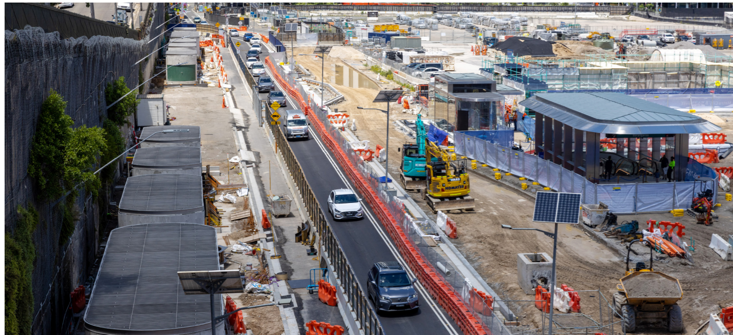
Barangaroo surface works
