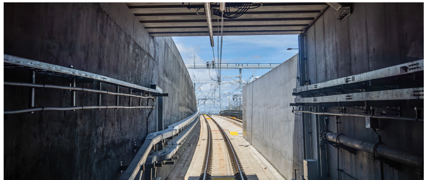
View from train exiting tunnel at Marrickville during testing
