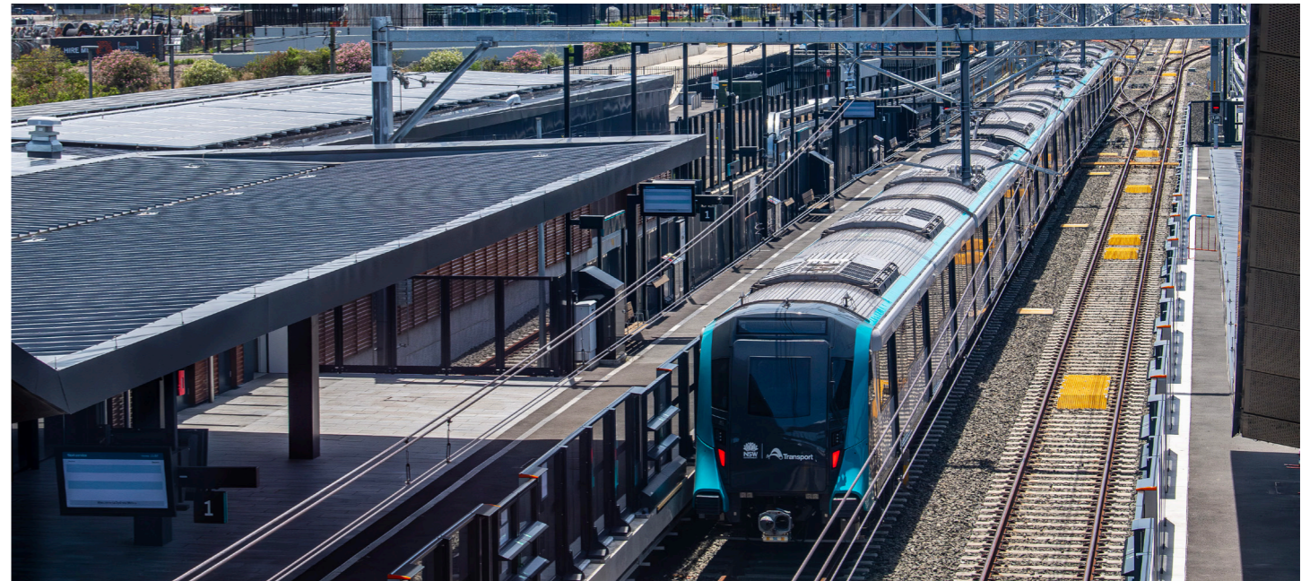
Train pulls into the new metro platform at Sydenham Station
