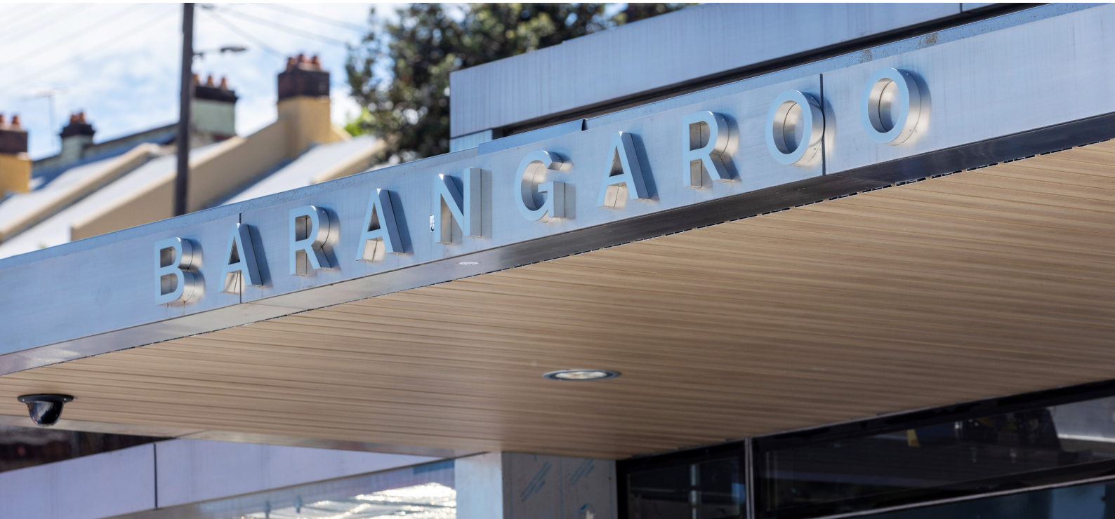
Barangaroo Station entrance canopy
