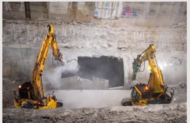
Multiple machines worked together to clear 230 metres of tunnel lining.
