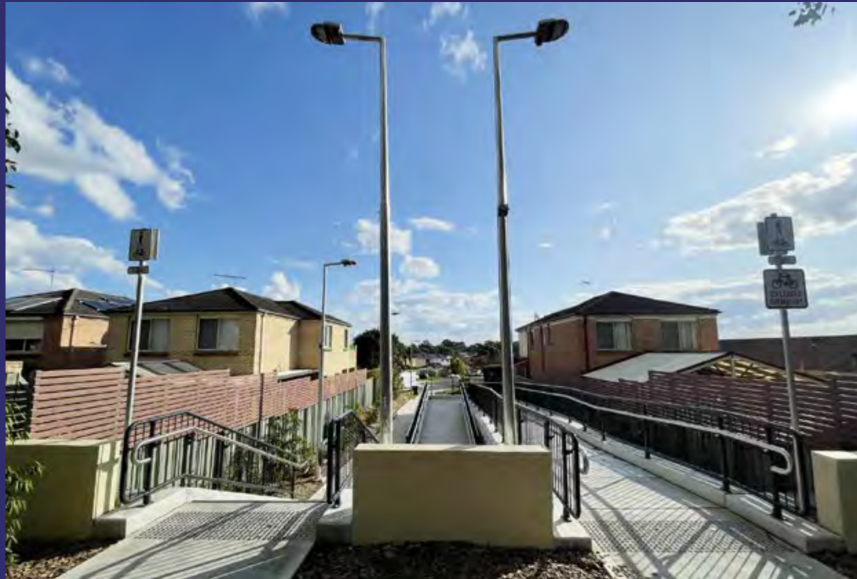
The new Glenwood Pedestrian Link.
