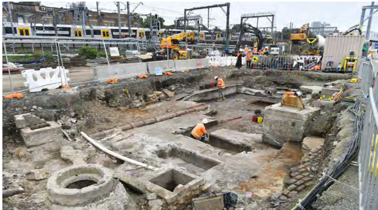
Excavation at Central Station.
