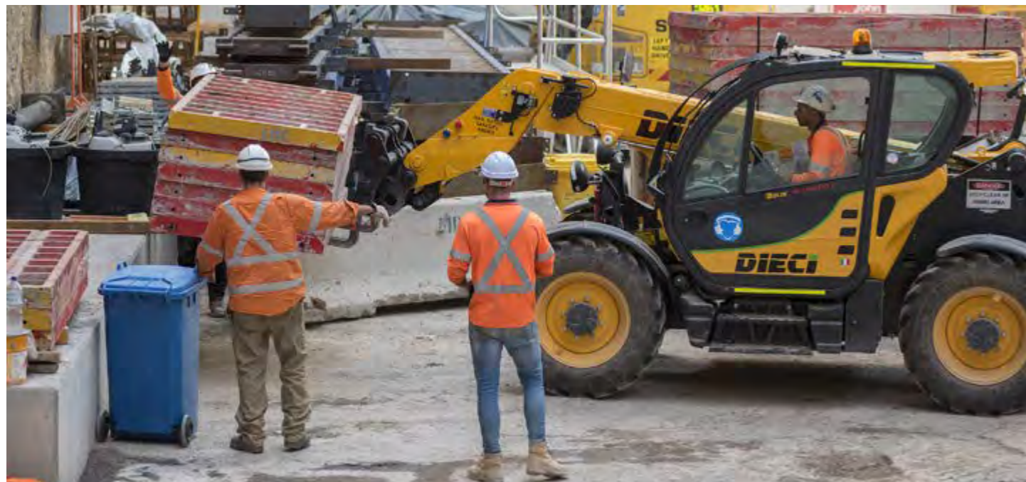
Materials storage at Bligh Street in Sydney's central business district.
