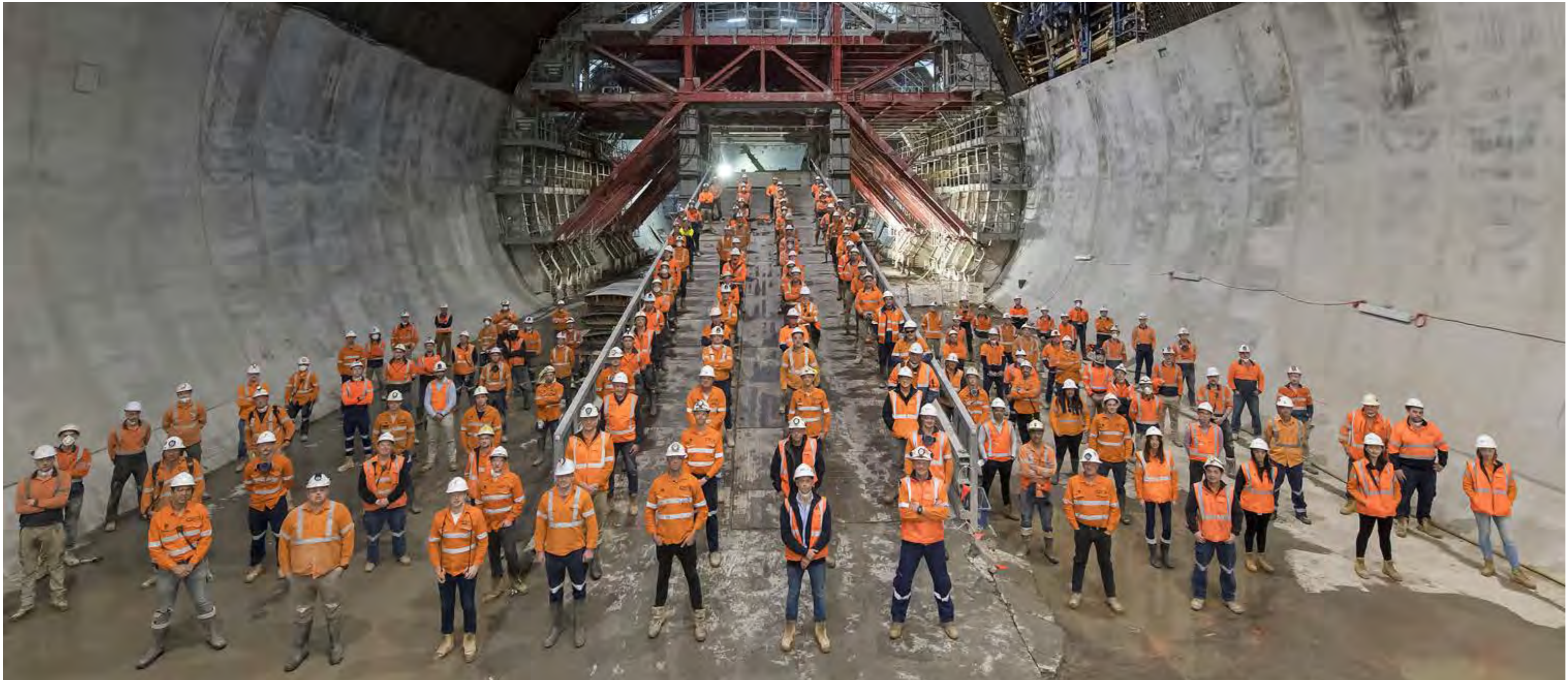
A team of workers about 31 metres underground at the Sydney Metro City & Southwest Victoria Cross Station, in the heart of the North Sydney business district.
