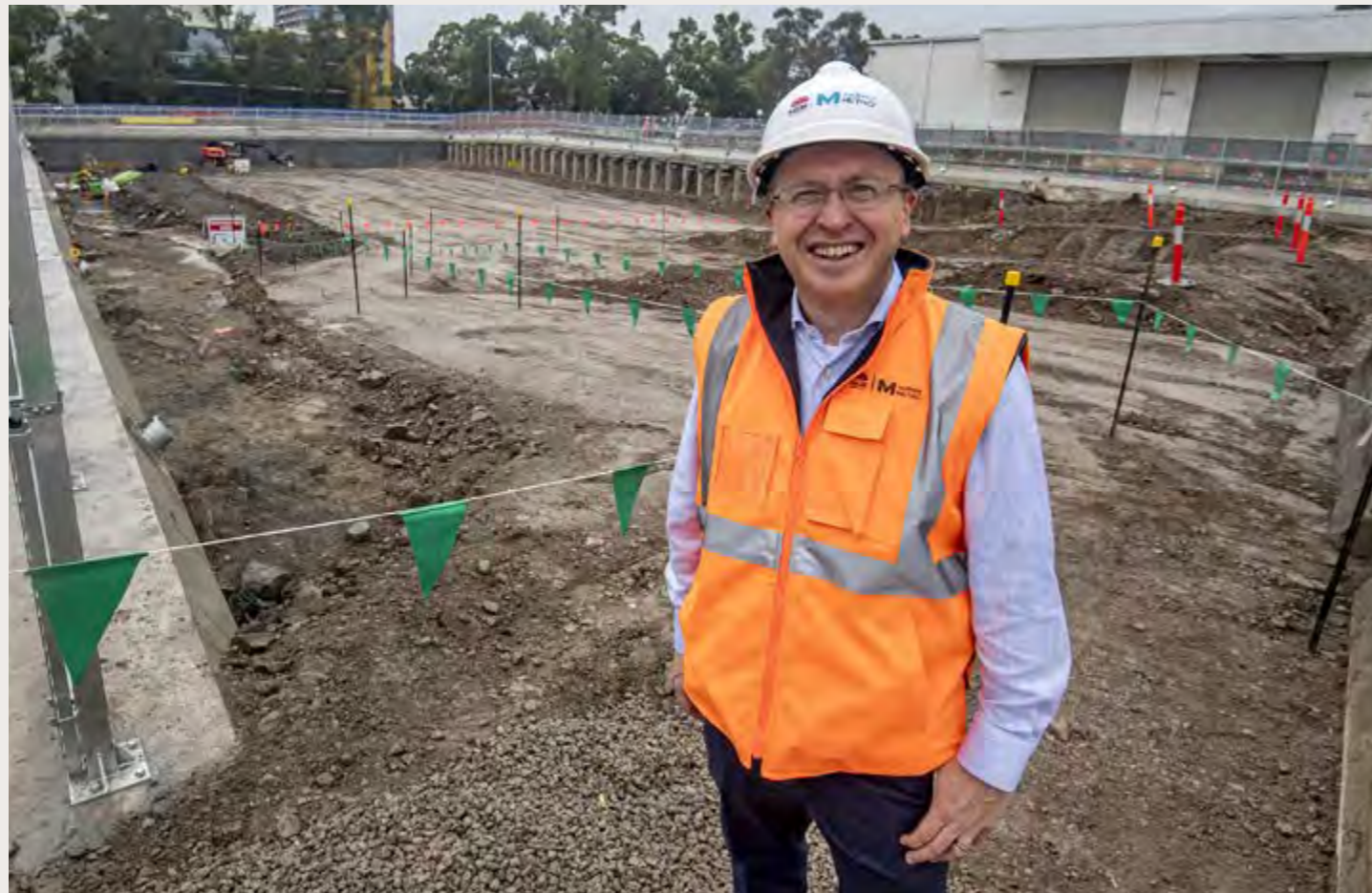
Peter Regan PSM, Chief Executive, Sydney Metro, pictured inside the station box at the Sydney Olympic Park Sydney metro station.
