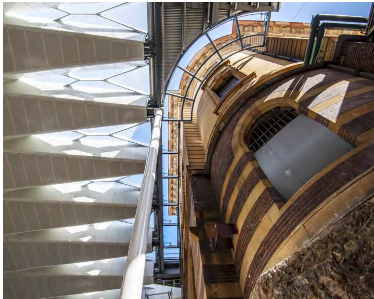
Northern Concourse at Central Station.
