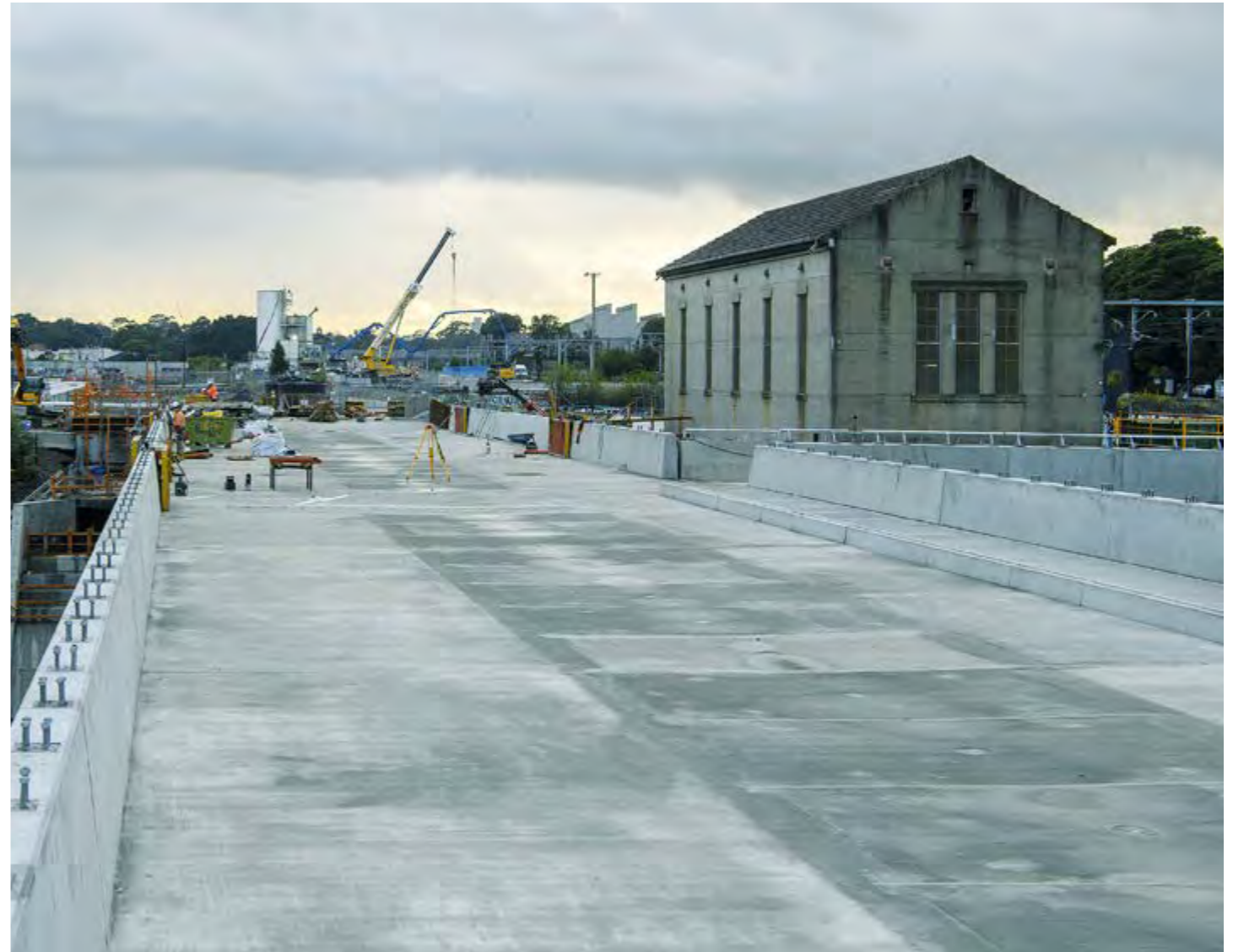
Construction of the new aqueduct over the existing heritage-listed Sydenham Pit, while retaining the existing heritage listed pump station.
