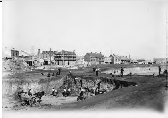
FIGURE 5.19: EXCAVATIONS FOR CENTRAL RAILWAY STATION WITH ELIZABETH STREET BEHIND. RAHS
