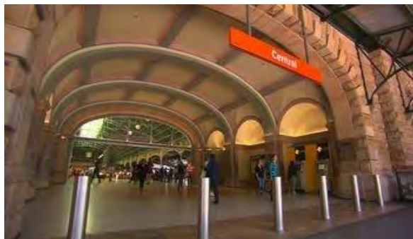
FIGURE 3.7: EXAMPLE OF A BANDED ARCHED PASSAGE THROUGH THE MAIN TERMINUS.
