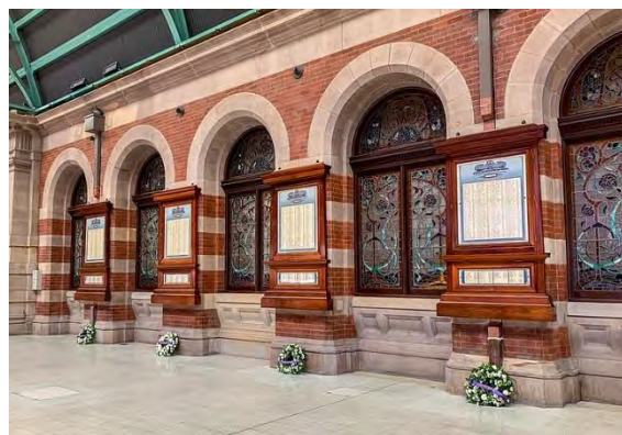
FIGURE 3.51: WWI HONOUR BOARDS CONSERVED AND REINSTATED IN THE GRAND CONCOURSE AT THE END OF 2018.
