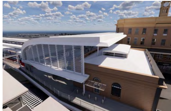
FIGURE 3.4: INTERPRETATION OF THE TRADITIONAL ARCHED FORM IN THE NORTHERN CONCOURSE CANOPY, WHICH INTERFACES WITH BOTH THE MAIN TERMINUS AND CENTRAL ELECTRIC BUILDING AS SHOWN IN THE IMAGE.
