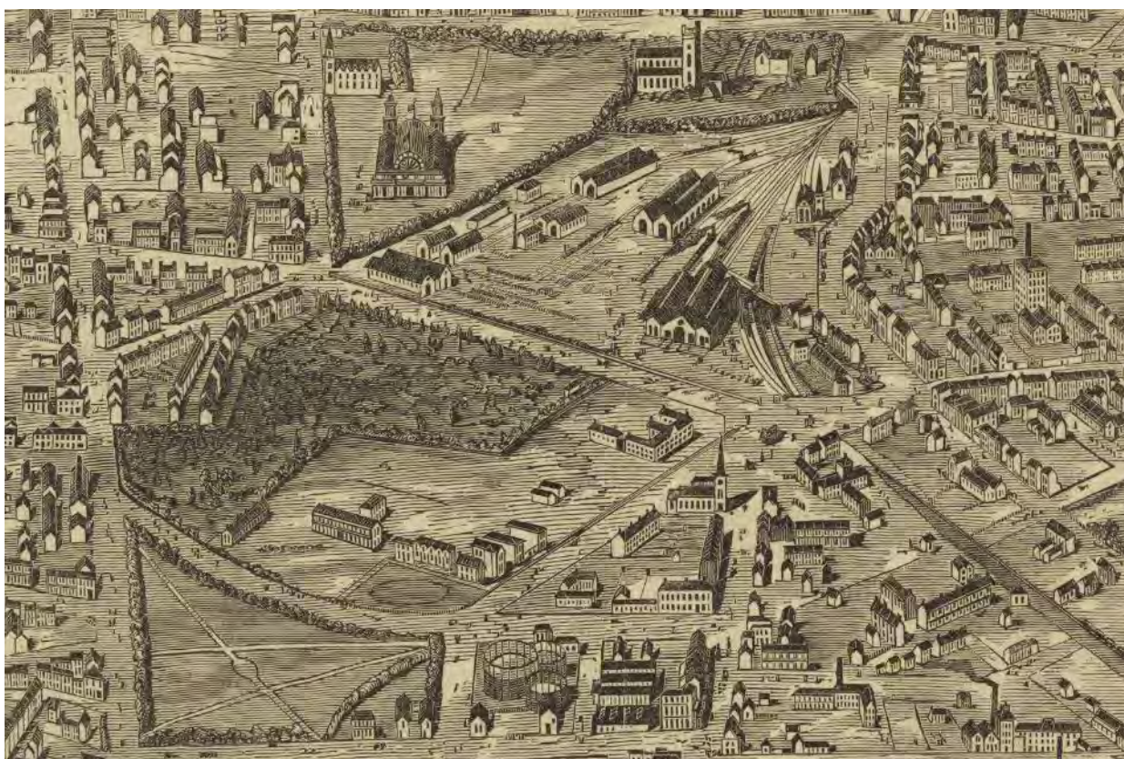
FIGURE 5.23: DETAIL SECTION OF WOODBLOCK CARVING PRINTED IN ILLUSTRATED SYDNEY NEWS, 1879, SHOWING THE SITE AREA OF THE CEMETERY AND THE SECOND SYDNEY STATION TO EACH SIDE OF DEVONSHIRE STREET.
