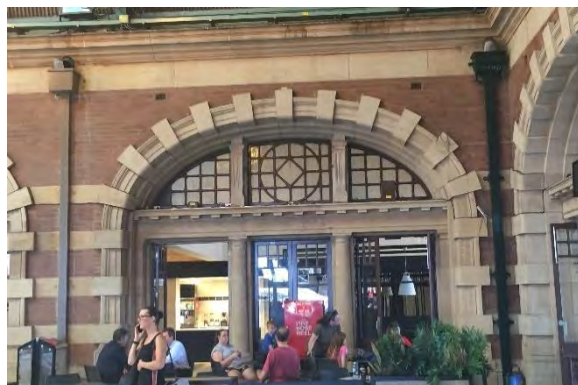
FIGURE 3.5: EXAMPLE OF WIDE ARCHED MASONRY OPENINGS PRESENT ON MAIN TERMINUS 'INTERIOR' FACADES FACING THE GRAND CONCOURSE.
