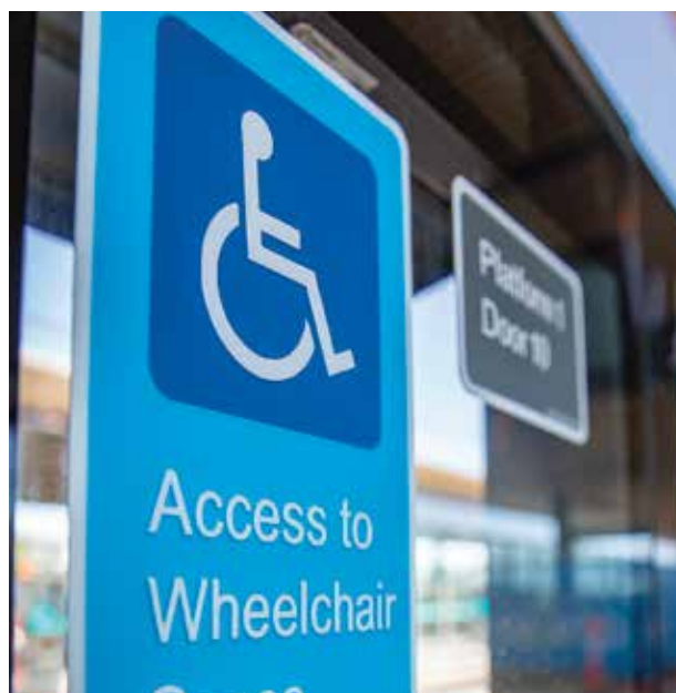
Wheelchair access sign on platform screen door.
