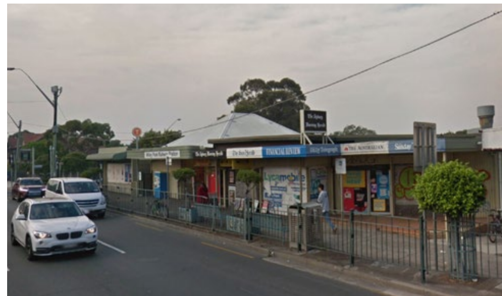
Figure 4.24 Existing condition of station entry and concourse
