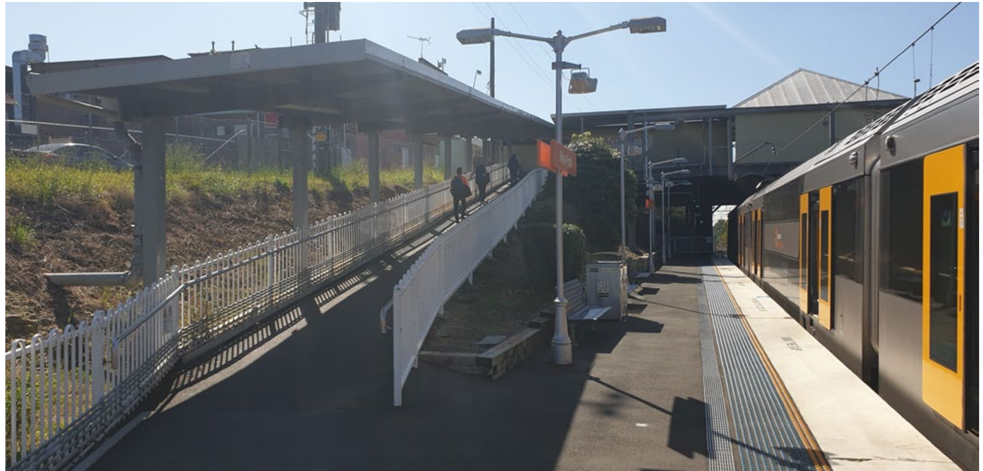
Figure 4.14 Existing ramps and canopies, platform 1
