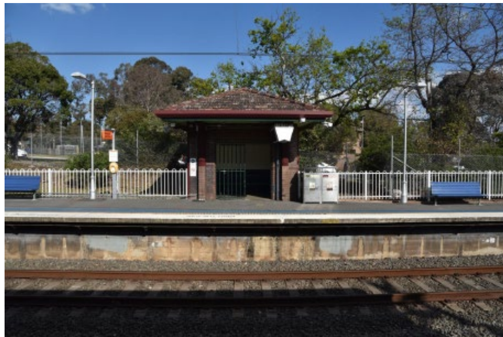
Figure 4.9 Existing waiting room current condition
