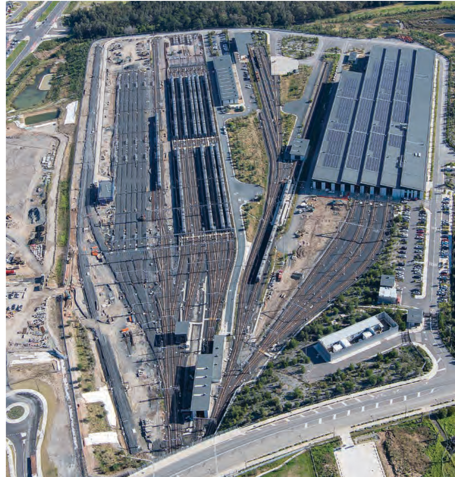
The Sydney Metro Trains Facility at Rouse Hill.
