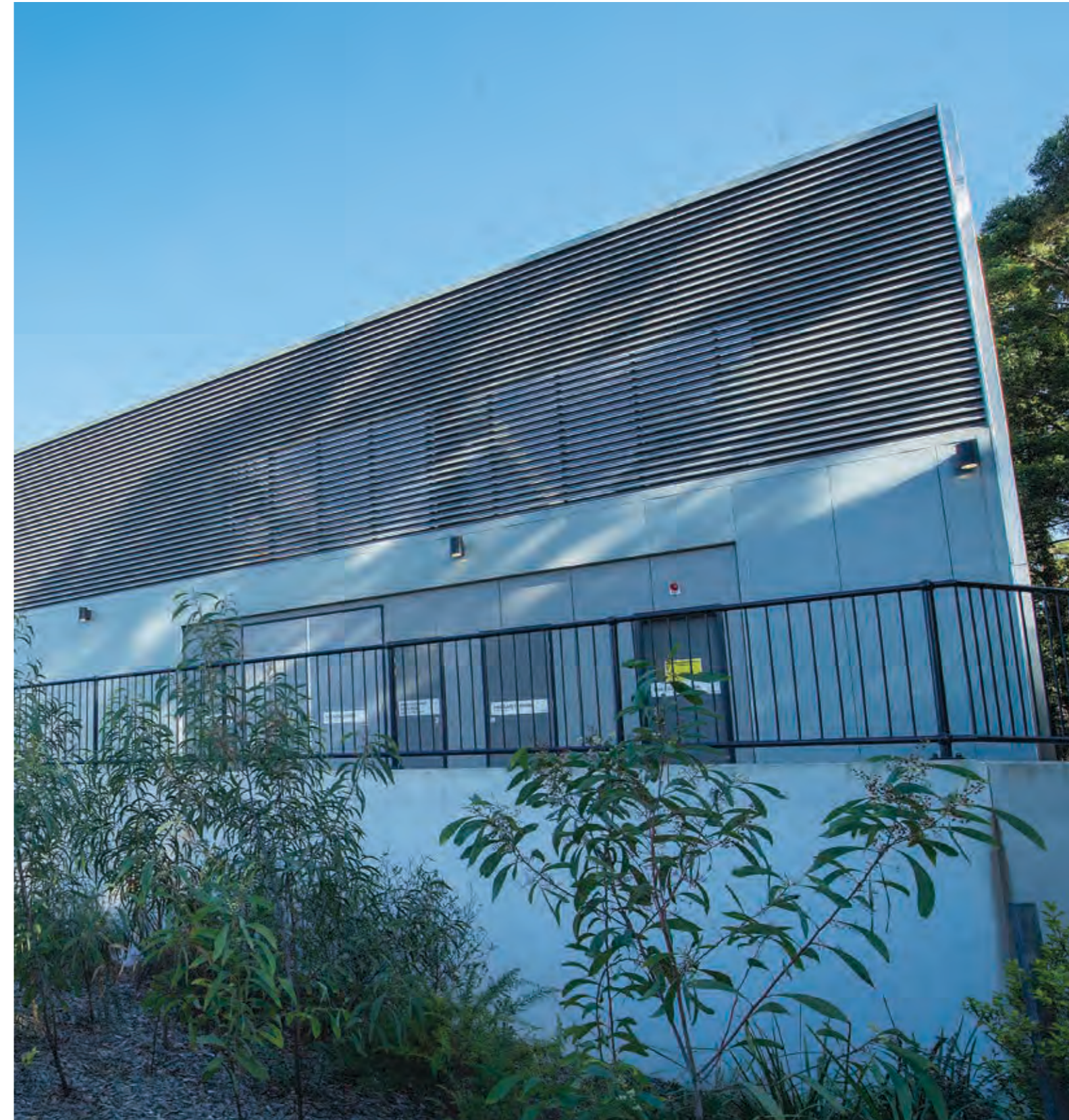
An example of a Sydney Metro services facility.
