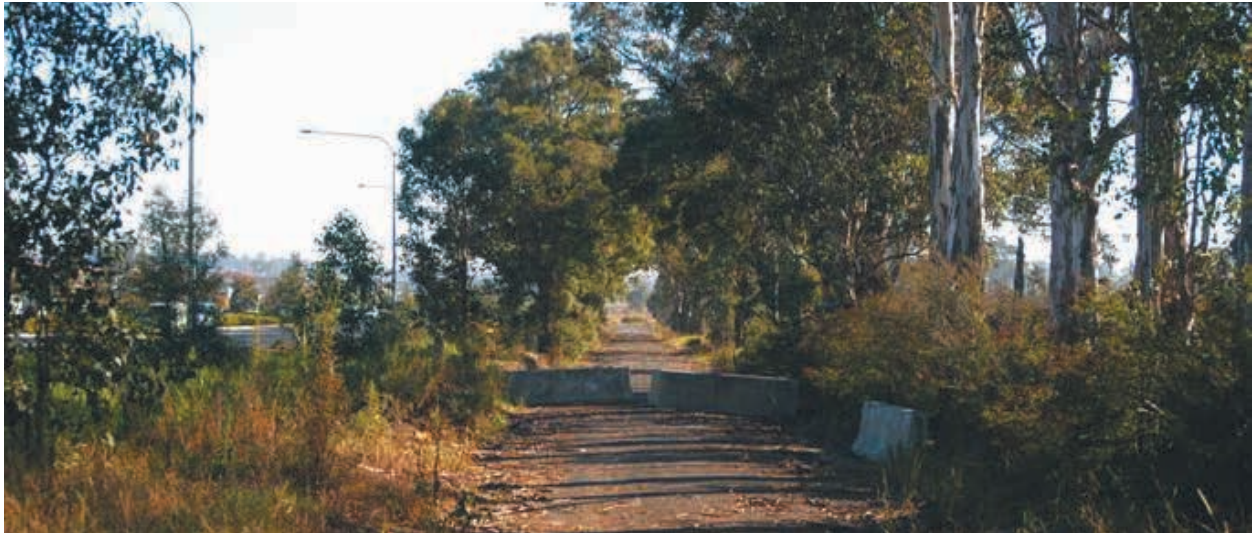
Figure 13: Remnant of the Old Windsor Road, Stanhope Farm alignment, Stanhope Gardens, Blacktown. Colonial roads were narrow, constructed of dirt and stone and lined with dense bush. Trees and scrub were later cleared as settlers moved into Sydney's west in search of farming land and commercial opportunities. NSW Office of Environment and Heritage http://www.environment.nsw.gov.au/heritageapp/ViewHeritageItemDetails.aspx?id=4301011 .
