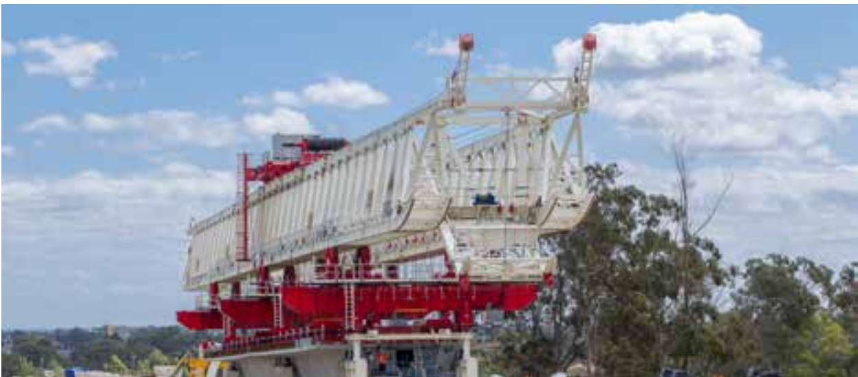
Figure 12: After the archaeological excavation began, it became clear that one of the piers for the viaduct design would impact the excavation site and the remains of the inn. The position of the pier was adjusted to conserve the site. https://www.sydneymetro.info/white-hart-inn
