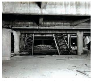
Figure 22: Wynyard Station: erecting the escalators, 1932.
