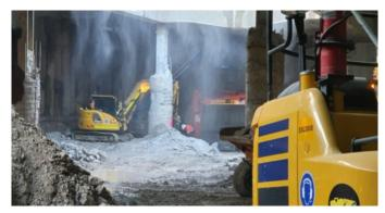
Misting system installed along the Metro Box.
