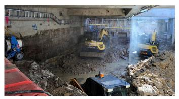
Canon misters used as a method of dust suppression during jack hammering works.
